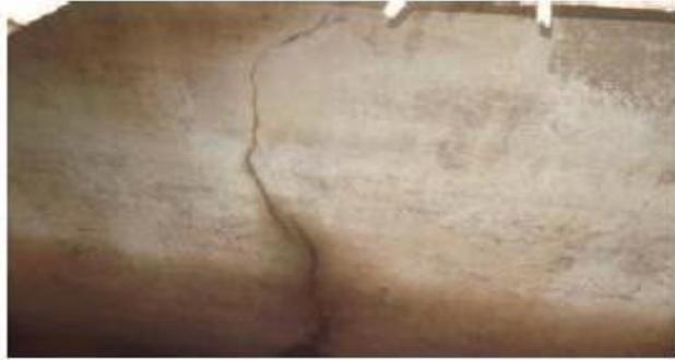
VISTA INTERIOR DONDE SE APRECIA LA GRIETA EN EL TANQUE.
